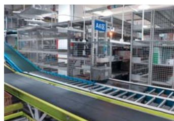
Conveyer belt at Jointown
